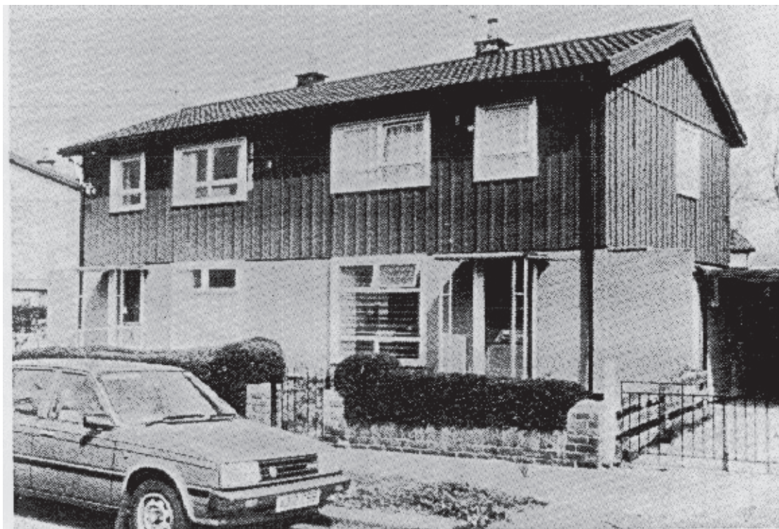
Figure 49: A typical BISF house
