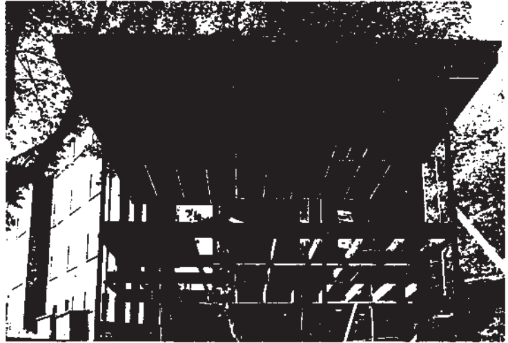
Figure 63: Flat roof frames on the Lewisham self build house (1980)
